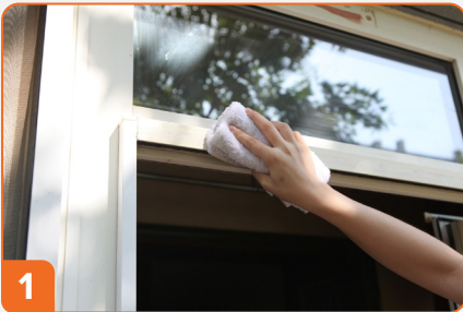
1 Clean door frame to remove any dirt or grease.
